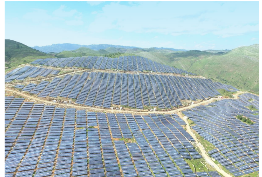
SolarMax Solar Farm Project in Guizhou Province, China
